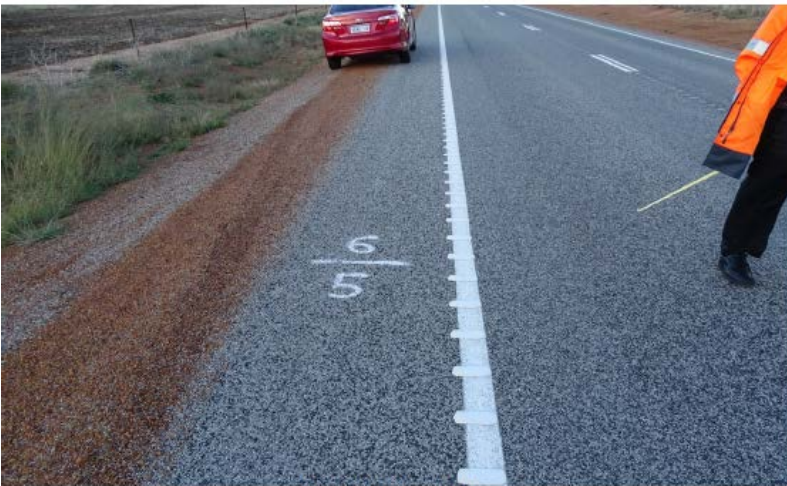
Figure B 37: Start of Trial Site No. 6 – edge of road
