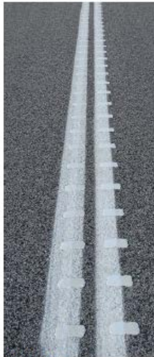
Centre Line Double Two-Way Barrier
