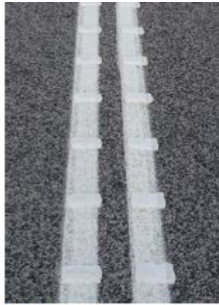
Centre Line Double Two-Way Barrier
