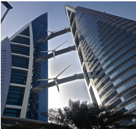
Image 6 -- baharian world trade Centre – first building integrated wind turbine generator
