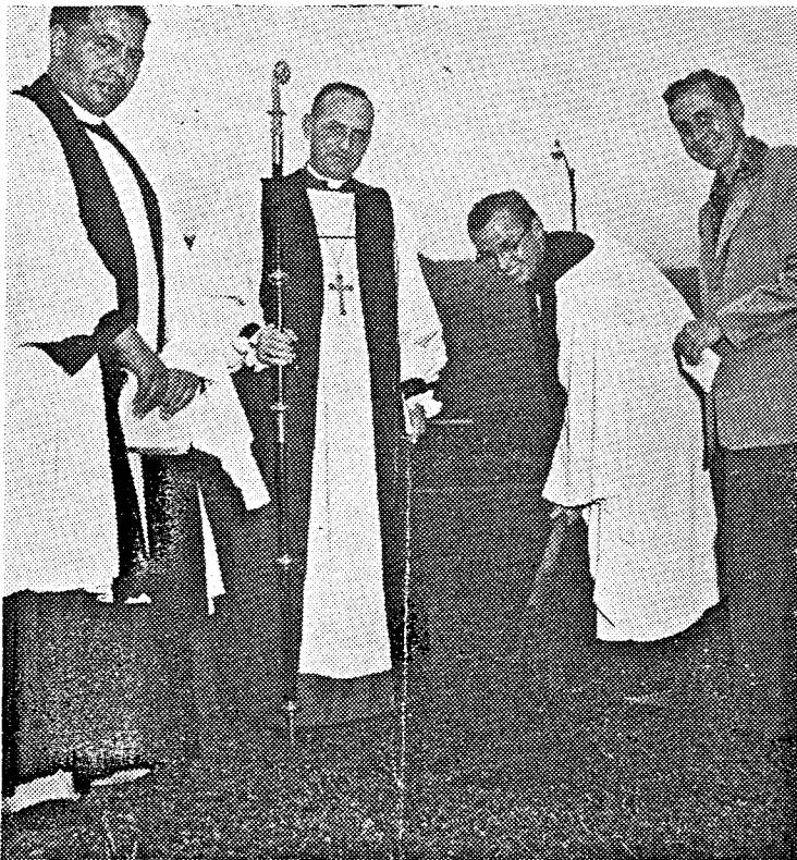
HOLY NATIVITY GROUNDBREAKING — Shown breaking ground are, left to right, the Rev. Manu Bennett, assistant vicar, Bishop Kennedy, the Rev. John J. Morrett, rector of the Church of the Holy Nativity, and Robert M. Law of the firm of Law & Wilson, architects for the new church.
