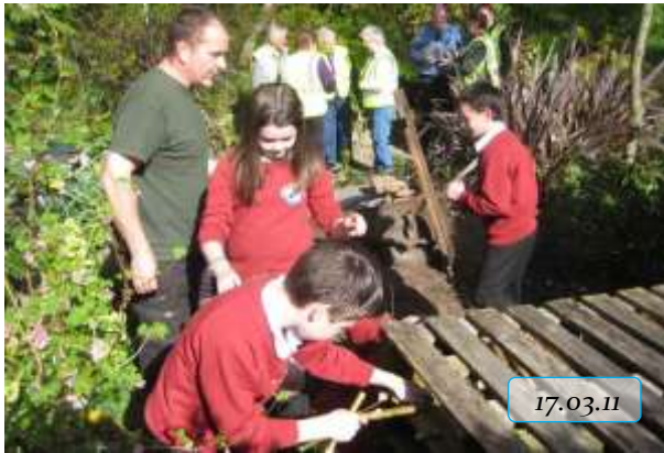
'Beast Mansion' under construction
