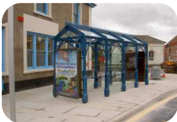
New Bus Shelter at Foundry
