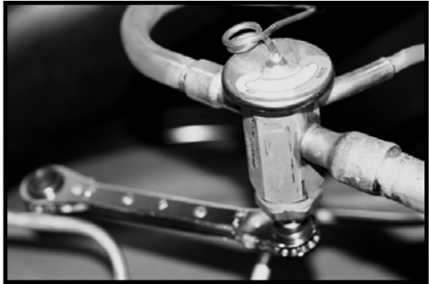
Adjust TXV with valve wrench
