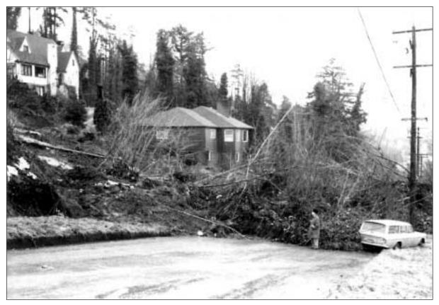
Figure 15. Unchannelized debris flow deposit.
