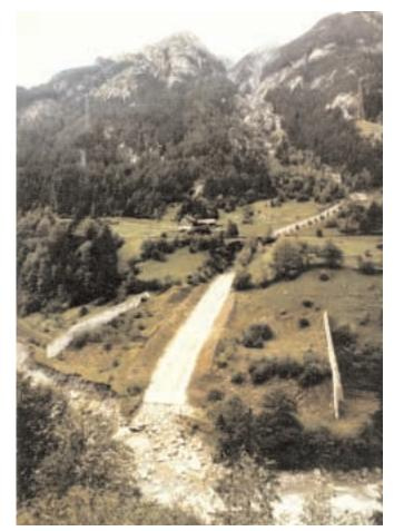
Figure 32. Steel-cell barrage structure set up on the Issyk River, Kazakhstan. (Photo from United Nations, 1996)
