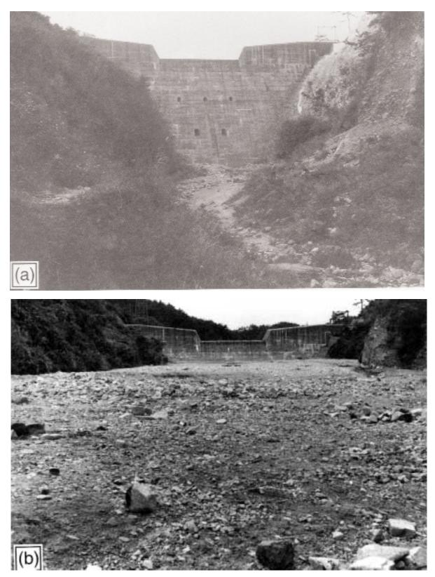
Figure 33. Check dam in Hyogo, Japan (30 m high, 78 m long, storage capacity 300,000 m<sup>3</sup>), (a) before and (b) after a debris flow. (Photo from United Nations, 1996)
