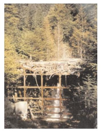
Figure 29. Steel-lattice dam constructed in Kirchbachgraben, Austria. (Photo from United Nations, 1996)
