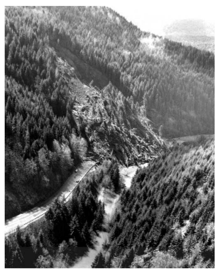
Figure 4. Rockslide that occurred along the Wilson River Highway (Hwy 6) in 1991. Though not a debris flow, this hazardous area is identified by the Further Review Area model. (Photo courtesy of Susanne L. D'Agnese, Oregon Department of Transportation)
