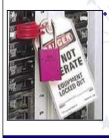
The Lock Out/Tag Out procedure prevents the unexpected start up or release of stored energy that could cause injury to employees by placing a lock and/or warning tag on an energy isolation device.
