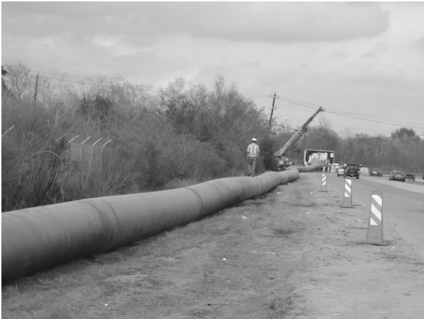
Figure 8. Pipe stringing and placement operations
