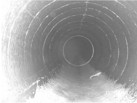
Circumferential cracks
