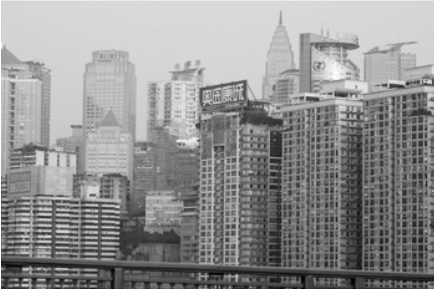
1 Construction boom in China (Chongqing) (David Legge)
