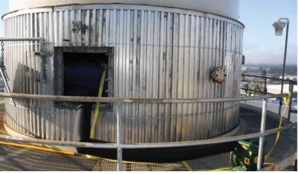
2. Typical stack balloon slopes toward the access for moisture drainage
