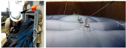
**6. Access door and platform** were added to accommodate the stack balloon (left); guy wire (right) holds the balloon during placement and is retracted during plant operation
