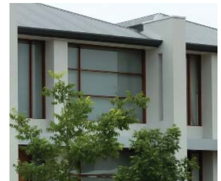
Timber framed windows
