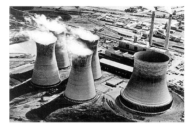
In the background: towers of the original plant for  $4 \times 200 \text{ MW}_{e}$  built in the 1970s In the foreground: cooling tower to serve 620 MW<sub>e</sub> supercritical extension (mid 1990)
