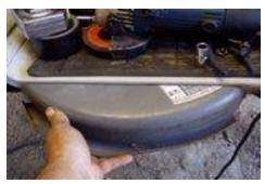
I hold it up to the running board and mark my line on each end so I know how much to cut off the bottom. I want it the same thickness of my running boards.
