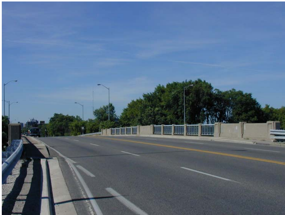
Plate 2. Christina Street Bridge deck looking south.
