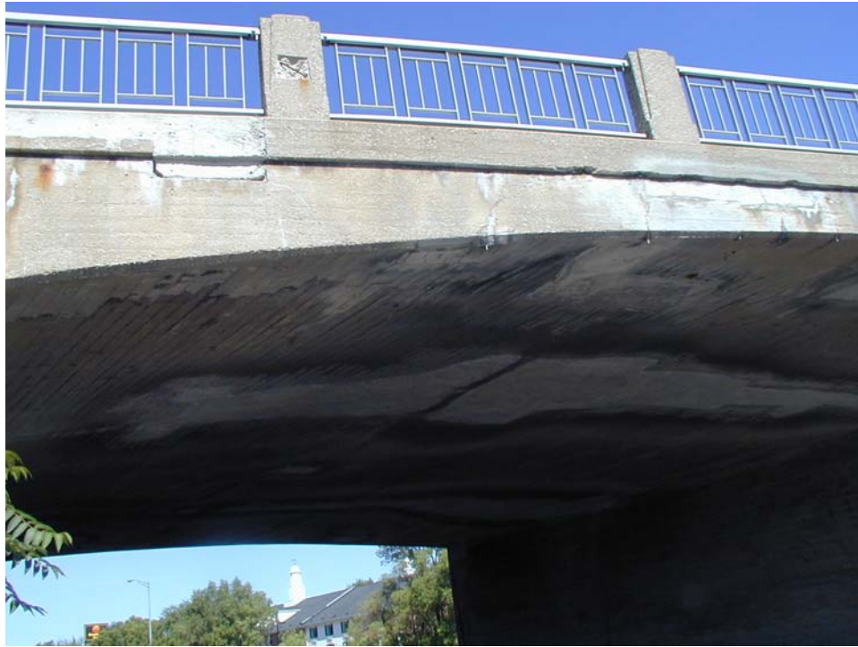
Plate 3. Soffit and railing.
