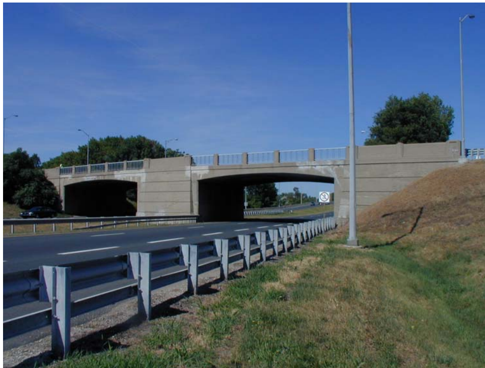
Plate 1. Christina Street Bridge over Highway 402, Sarnia, Ontario.
