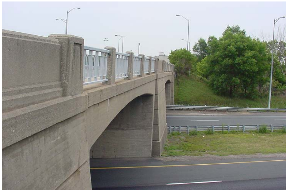
Plate 4. West elevation detail
