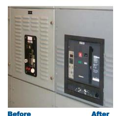
**Passive** components (bus, terminals, structure) remain while replacing *active* components
