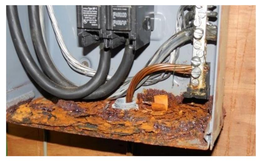
• Internal corrosion conditions occur undetected unless routine inspections are implemented
