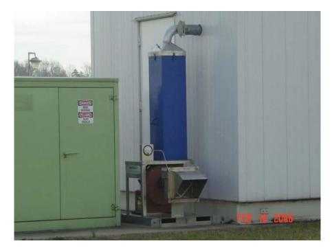
Where unable to locate electrical equipment in "clean" areas then consider mitigating corrosive gas penetration
