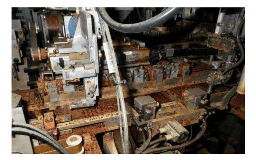
Corrosion can affect protective equipment clearing time including "no trip" failure mode
