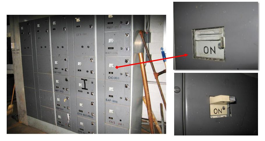
"Circuit breakers should be cycled ON-OFF at least every 6 months" – ANSI/NEMA AB 3
