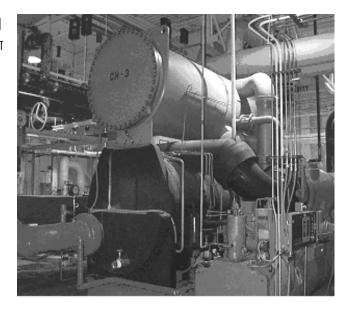
Chiller energy can account for 10 to 20% of total cleanroom energy use. The majority of annual chilled water use goes to medium temperature chilled water requirements  $-55^{\circ}$ F for sensible cooling and 60 to 70°F for process cooling loads. When outside air temperatures are cool and humidity is low (i.e., no low-temperature water is needed for dehumidification), 100% of the chilled water is for medium temperature loop uses.
