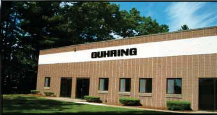
Connecticut Reconditioning Facility 121 W Dudley Town Rd. Bloomfield, CT 06002 Tel (860) 216-5948 Fax (860) 519-5819
