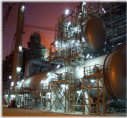
World's largest SRU Tail Gas Incineration System (Qatar). One of 9 similar incineration systems supplied by Zeeco.
