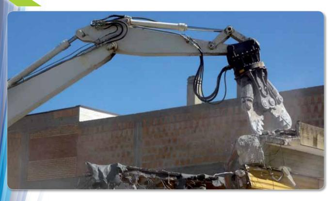
The field of **demolition** represents one of the main applications of pressure intensifiers. In this field, the weight of the cylinders linked to the demolition crusher, permits more extension of the operating machine arm they are connected to. The use of an intensifier allows reducing the cylinder diameter or employing crushers with a higher closing force.
