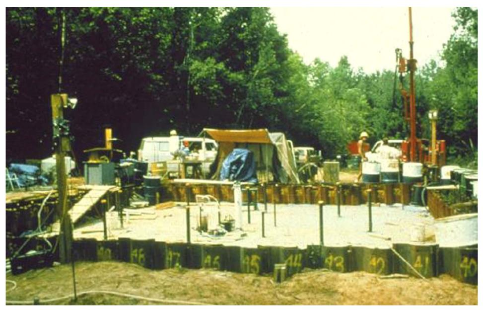
Double Wall, Sealable Joint Sheet Piling Cell Keyed into Aquitard
