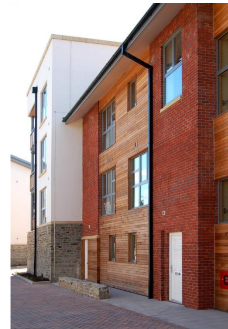
Figure 23: Timber Cladding (Combustible) (© Courtesy of Arup)
