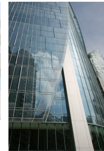
Figure 26: Glazing (non-combustible) (© Courtesy of Arup)
