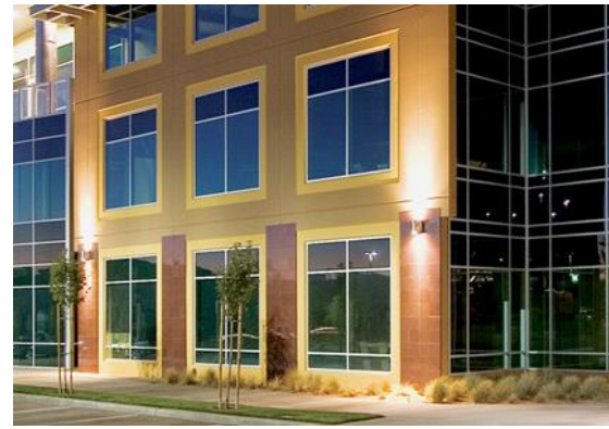
Figure 28: Lights on external façade (© Courtesy of Arup)
