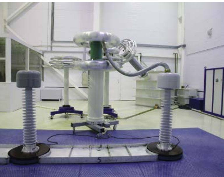
Fig. 15. Electrical tests of 126 kV bushings at the Izolyator plant
