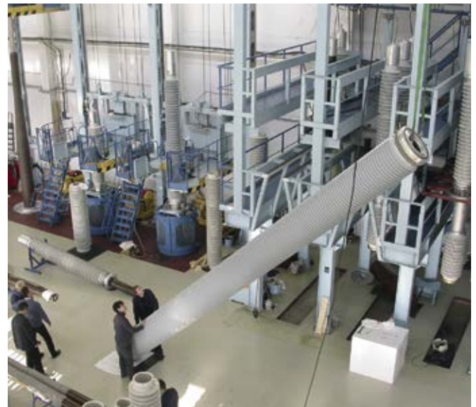
Assembly of extra-high voltage bushings in Izolyator factory
