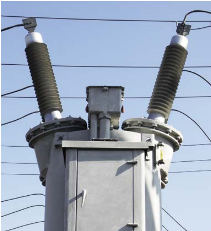
Bushings 126 kV produced by Izolyator company on the oil switch of an inter-regional distribution grid company
