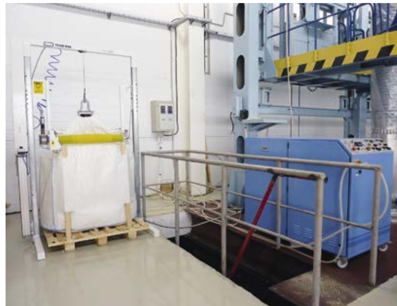
Fig. 12. Unit for degassing and metering feed of compression gel at the Izolyator plant
