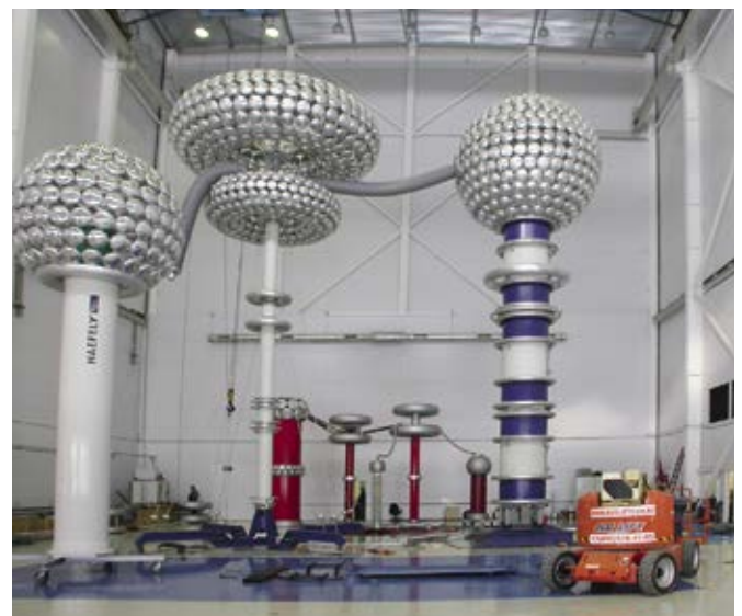
Testing Center of Izolyator factory
