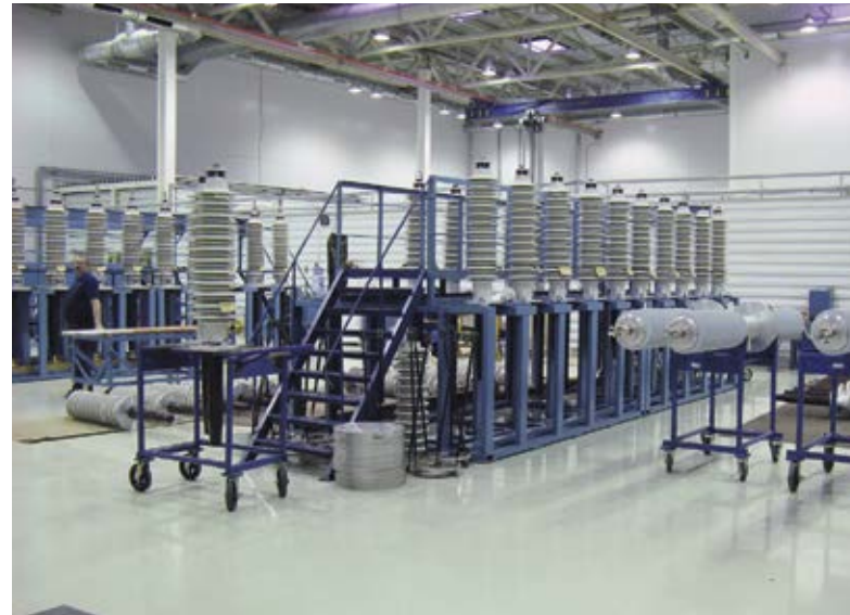
Fig. 11. 40.5-172 kV bushing assembly area at the Izolyator plant
