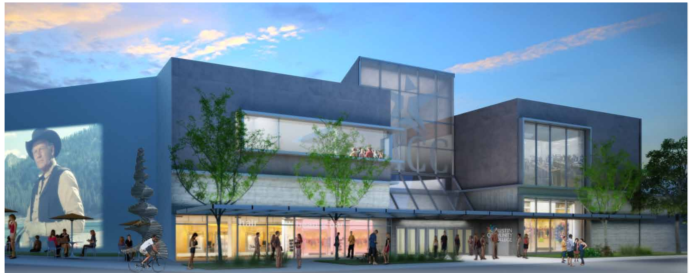
View of South Entry (formerly Macy's) and adjacent courtyard. Digital projection technology turns a solid facade into a large-scale projection screen that can be used for movies, artwork/digital murals or projections of performances being held in performing arts venues.
