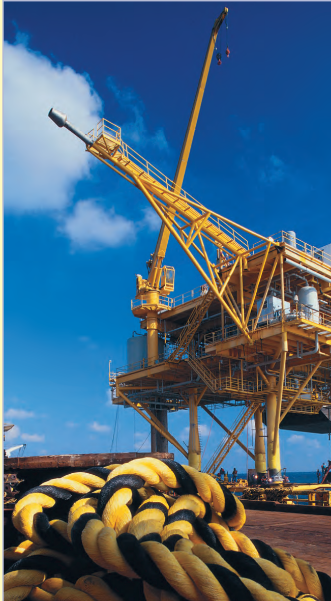
Floating drilling unit for offshore use
