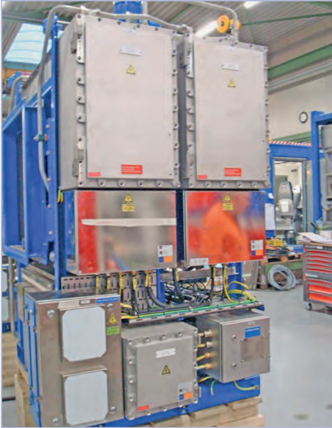
Figure 14: Power pack container (in progress), compact design
