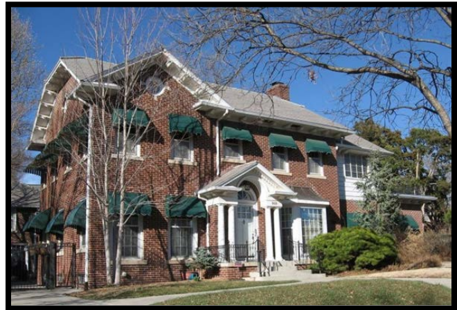
FIGURE 35: APPROPRIATELY SIZED AND PLACED AWNINGS.
