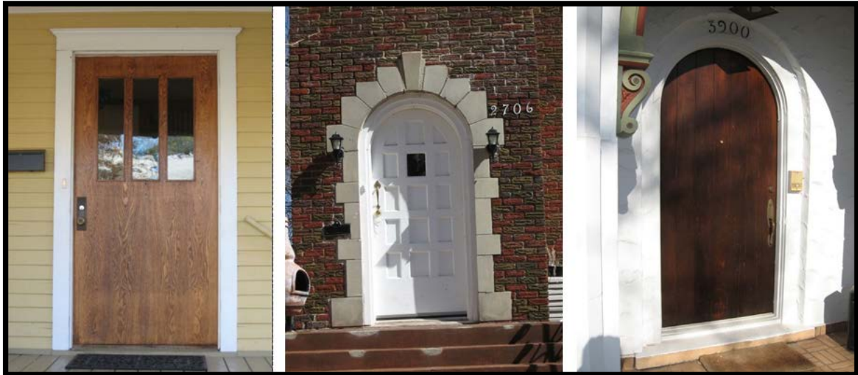
FIGURE 28: CHARACTER-DEFINING DOORS: CRAFTSMAN STYLE, LEFT; ARCHED TUDOR REVIVAL STYLE, CENTER; ARCHED SPANISH COLONIAL REVIVAL STYLE, RIGHT.
