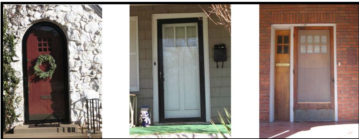
FIGURE 29: A STORM DOOR ADDED ON FRONT FAÇADES SHOULD BE A FULL-VIEW DESIGN AND FIT THE DOOR OPENING.
