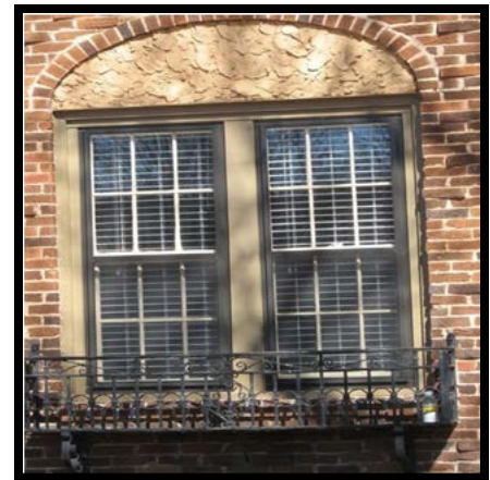
FIGURE 33: STORM WINDOWS SHOULD BE FULL-VIEW DESIGN OR HAVE STRUCTURAL FRAMEWORK ALIGN WITH WINDOW MEETING RAIL (PICTURED).
