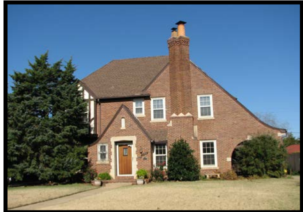
FIGURE 11: EXAMPLE OF THE TUDOR REVIVAL STYLE, 723 N.E. 21ST ST.
