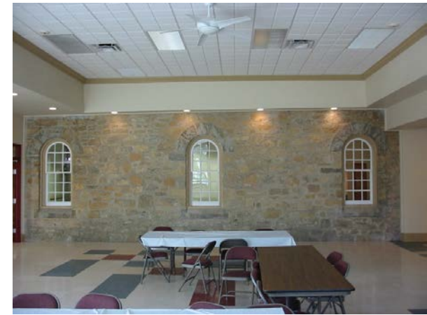
fellowship hall with exterior chapel wall
