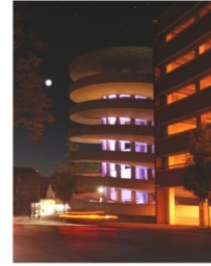
Prince Street Garage Helix
