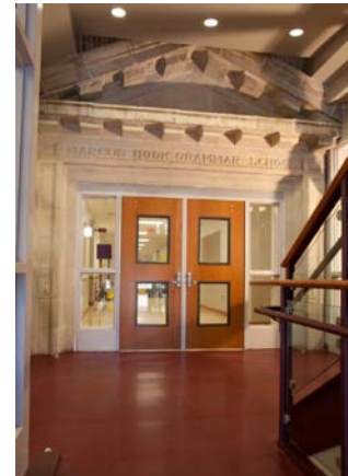
historic pediment on new main entry vestibule
