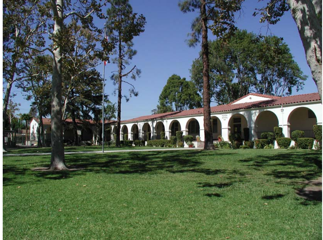
Los Angeles Unified School District Facilities Services Division Reseda Elementary School Opened in 1916
