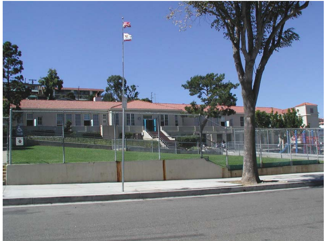
Los Angeles Unified School District Facilities Services Division Point Fermin Elementary School Opened in 1912
