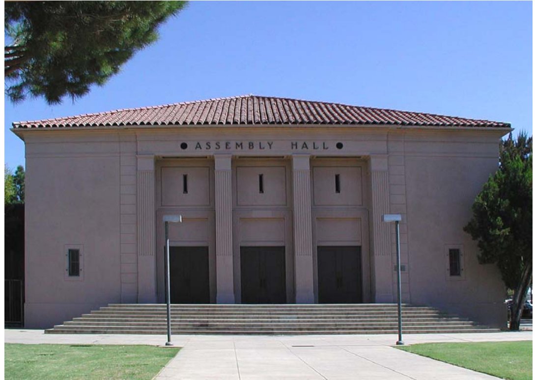
Los Angeles Unified School District Facilities Services Division Canoga Park High School Annexed in 1915
