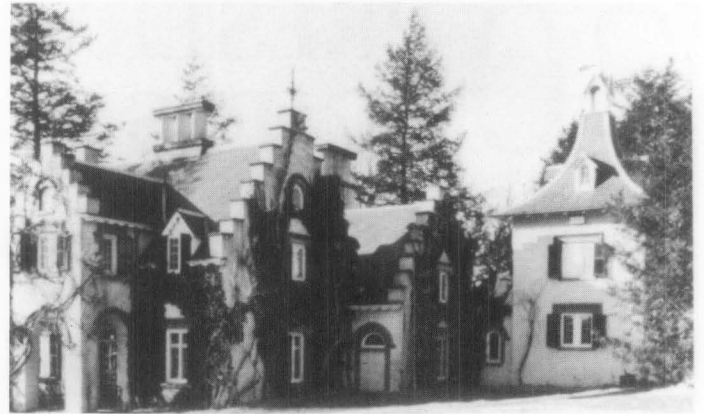
Fig. 2. Sunnyside, Washington Irving's house in Tarrytown, New York, dates to about 1656. Although extensively remodeled during the years 1836-1849, the stepped gables and tiled roof still reflect the heritage of its original Dutch builders. Photo: Jack E. Boucher, HABS Collection.
