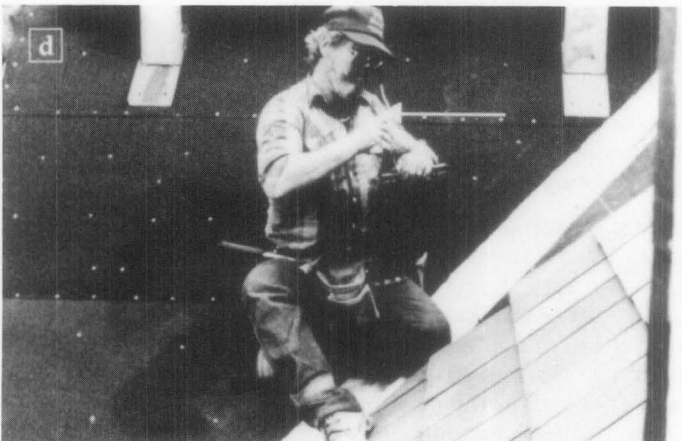
Figure 12. When constructed in Frankfort, Kentucky, in 1900, the Colonial Revival-style Berry Hill Mansion, and its 1912 Music Room addition were both roofed with "Imperial" tiles manufactured by Ludowici-Celadon (a). In 1992 the entire roof was replaced because of deterioration and surface spalling of many of the tiles (b). It was not possible to reproduce the original tiles due to budget limitations, thus Ludowici-Celadon's stock "Classic Interlocking" Shingle tiles were selected as replacements which could provide a close, if not exact, match. After tearing off and removing the old tiles, 30 lb. roofing felt was laid over the existing wood sheathing, new lead gutters and valleys were installed, and 90 lb. roll roofing was laid, on which the new tiles were laid. Although most of the field tiles were simply attached by 2 nails to the substrate (c), many of the tiles that had to be cut to fit hips, valleys and dormers were left with only one hole, and had to be wired and then nailed in place (d-e). The exact color and glaze of the original tiles also could not be duplicated because the coloring material is no longer available; however, the new hipped roof terminus for the Music Room roof was custom-made and the replacement field tiles are very similar to the originals (f). The original ridge tiles were designed to "nest" and fit perfectly over the field tiles beneath them whereas the new ridge tiles simply overlap one another, but this is barely perceptible when viewed from the ground. Photos: Edwin C. Krebs, AIA.
