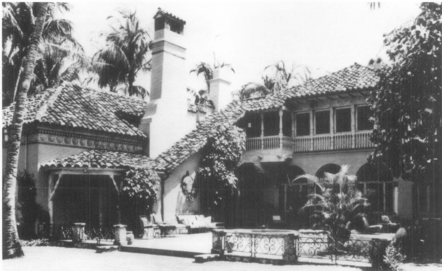
Fig. 6. Like many other house of this period in Florida, the roof of the Chester C. Bolton House in Palm Beach features tiles imported from Cuba. These tiles, with their richly varied earth colors, were often laid in thick cement mortar that was intended to give a "rustic" appearance. The residence, which includes the main house (1918-1919) designed by James A. Garfield, and an addition built in 1929 designed by Prentice Sanger, has been described as an English manor house with Spanish details. Photo: Jack E. Boucher, HABS Collection.
