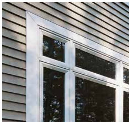
Charter Oak clapboard with Trimworks 5" window trim.
