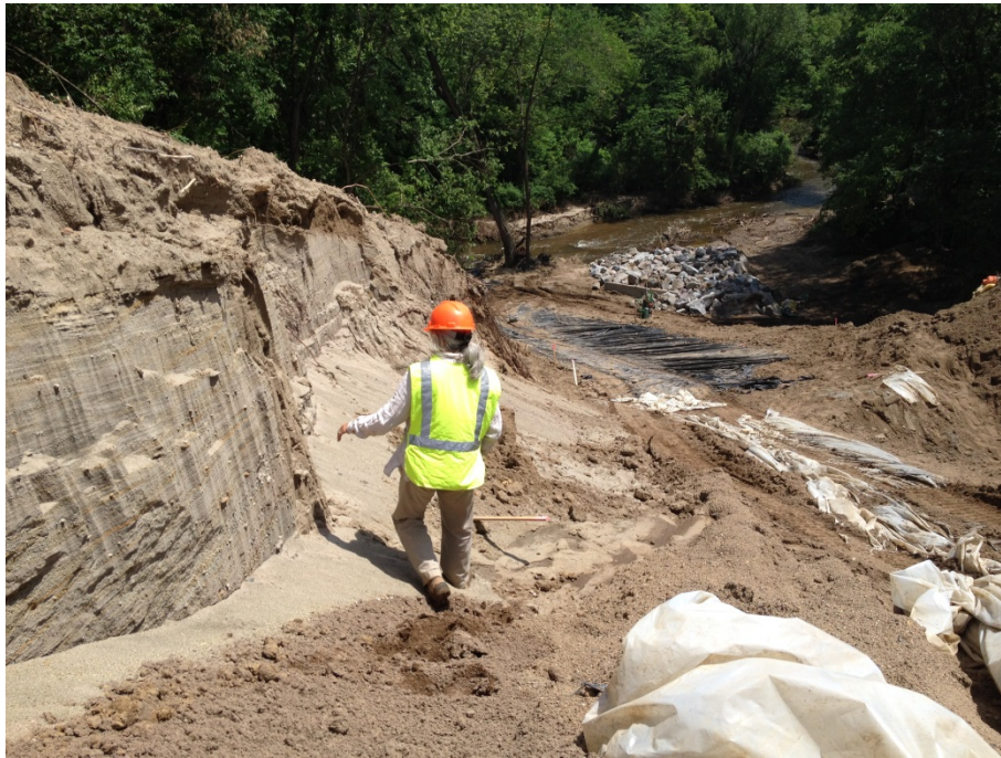
Figure 13. Dry sand and gravel slopes in Eden Prairie undergoing repair.
