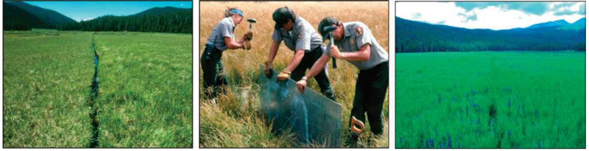
Figure 43 —Ditch in Big Meadows, Rocky Mountain National Park in 1989 (left panel), prior to hydrologic restoration by National Park Service personnel using sheet metal check dams (center panel). The same area in 2006 (right panel) (photos: D. Cooper).
