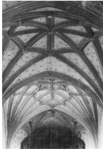
Ribbed vault diagram and photo of ribbed vault
