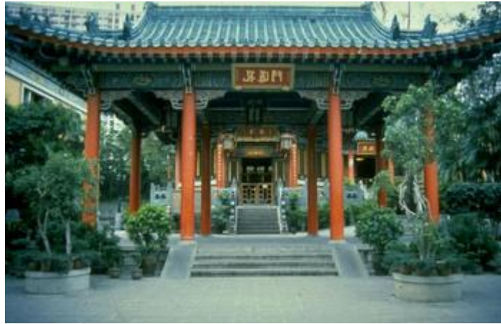
Pagoda columns, roof
