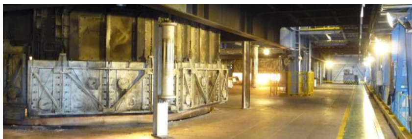
Figure 11: FeSi furnace of POSCO during operation
