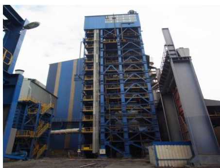
Figure 7: Energy recovery system under construction for Etikrom
