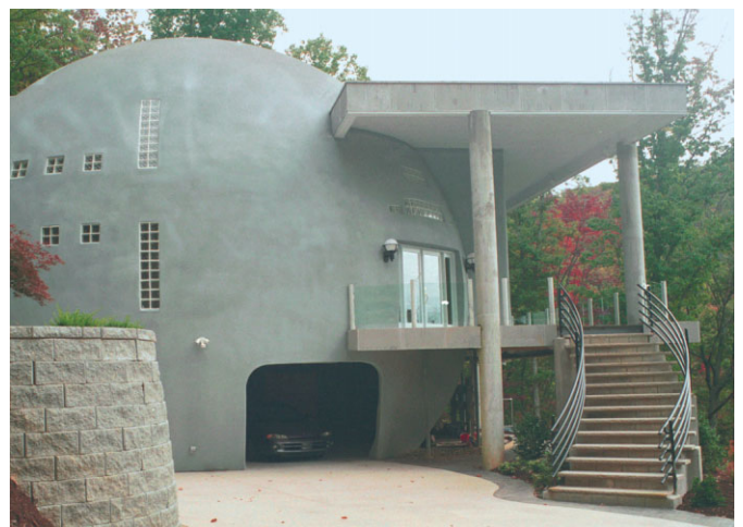
Fig. 18. Cloud Hidden house, built using pneumatic formwork (2000). Reproduced by permission of the Monolithic Dome Institute
