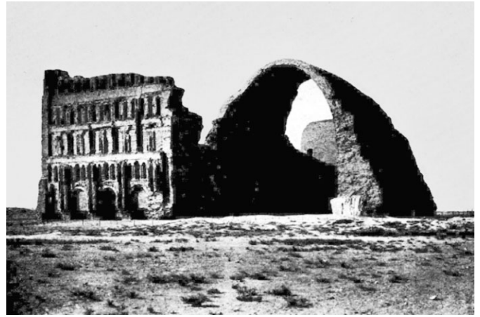
Fig. 6. The ruins of the Taq-i Kisra palace at the ancient city of Ctesiphon [9]
