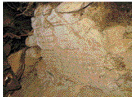
Fig. 1. Impressions of reeds in the vault of a channel near Menacer, Algeria. Reproduced by permission of Cees Passchier
