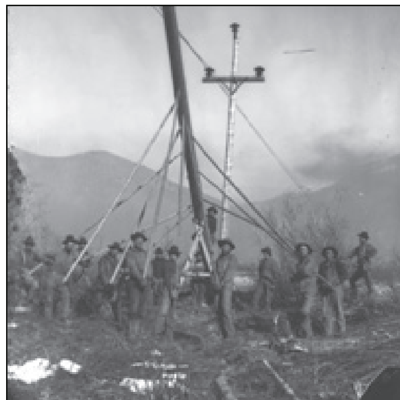
A crew raises an electrical pole by hand in this undated photo from the archives of the La Plata Electric Association. Courtesy of LPEA
