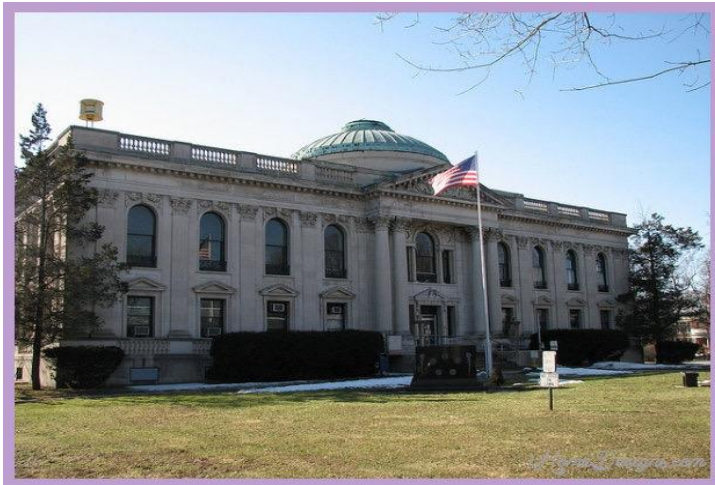
Columbia County Courthouse, present day
