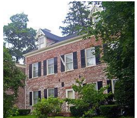
Elisha Williams House in Hudson (1810), National Register of Historic Places
