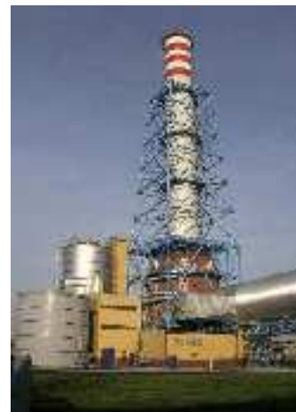
Koziernice II Project 800MW (Poland)
