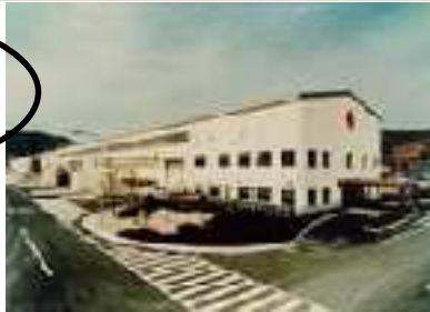
BHK Catalyst Manufacturing Facility in Japan (Akitsu Works)
