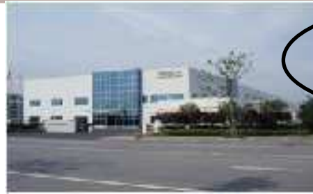
BHK Catalyst Manufacturing Facility in China (BHHE)
