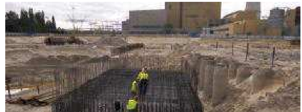
Construction status as of September 2013
