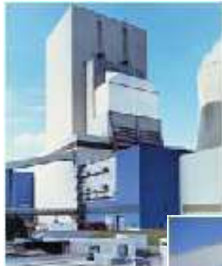
Germany, Mehrum No.3 700MW, Coal
