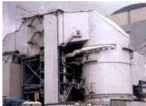
Tachibanawan No. 2 1,050MW (Japan)
