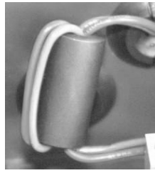
Figure 2-5: Ferrite core and battery supply wiring
