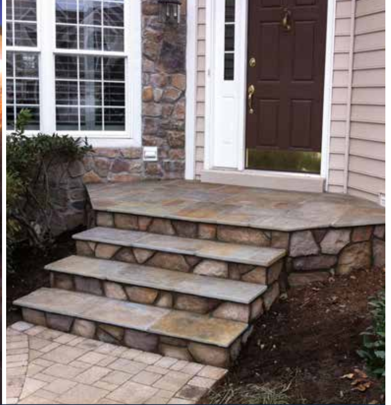
FLAGSTONE OVERLAY STOOP WITH HOLLOWAY FIELDSTONE VENEER AND PAVER WALKWAY.
