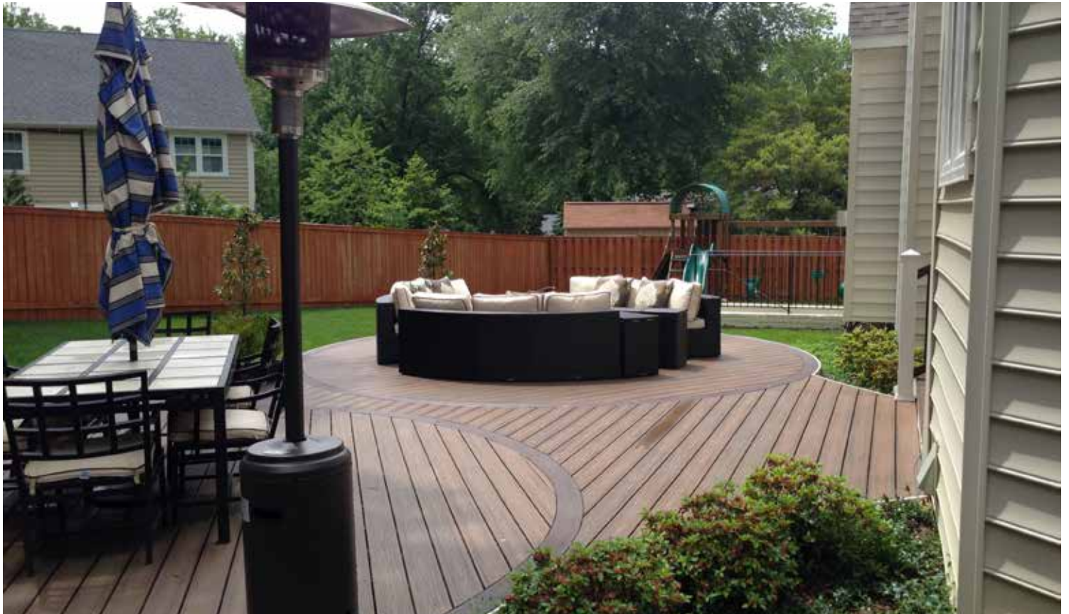
ABOVE: TREX TRANSCENDS DECKING: SPICED RUM WITH VINTAGE LANTERN BORDERS. DECK HEIGHT IS BELOW 30" FROM GRADE THEREFORE NO RAILS NEEDED.
