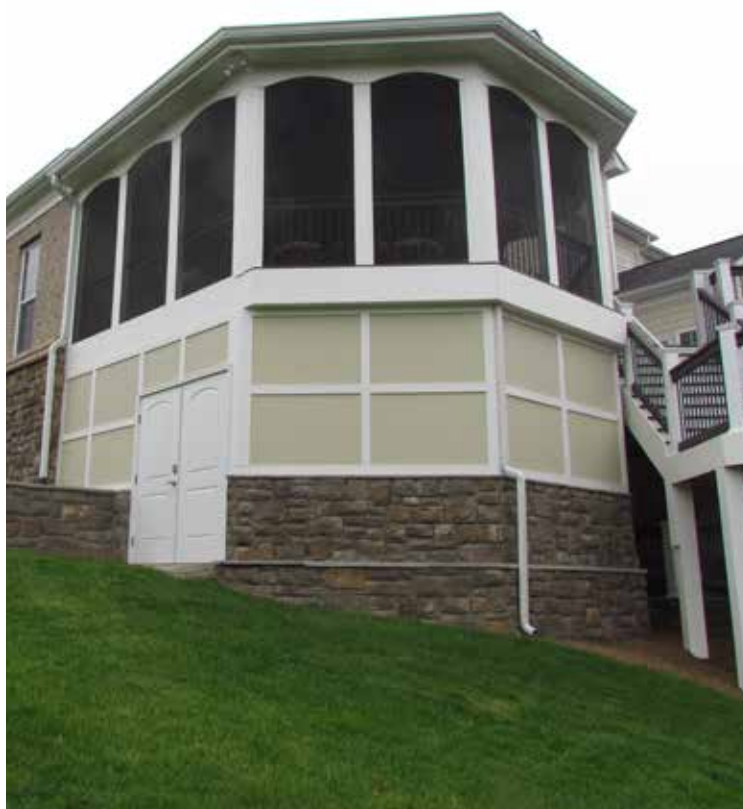
ABOVE: EXTERIOR VIEW OF SCREEN-TIGHT SCREENED PORCH. STORAGE BELOW WITH WHITE TRIM, HARDIE-BOARD AND CULTURED VENEER.
