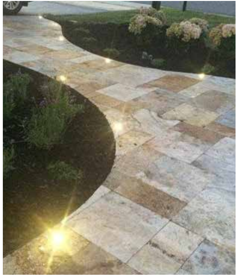
TRAVERTINE (SCABOS) IN DRY BASE WITH EMBEDDED ACCENT EDGE LIGHTS.
