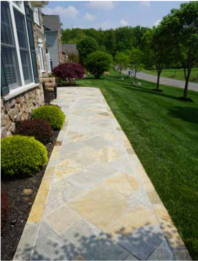
PATTERN FLAGSTONE IN CONCRETE BASE WITH MORTARED JOINT.
