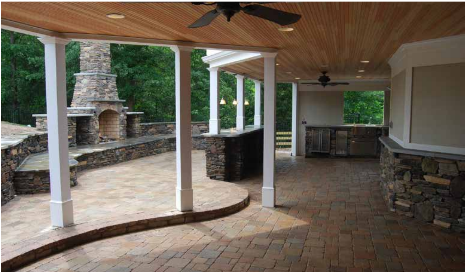
ABOVE: CUSTOM DRY SPACE WITH NATURAL BEADED FIR CEILING, LIGHTING, PVC WRAPPED POSTS AND BEAMS, VENERED WATER-TABLE WITH LEDGE BUFFET, SERVING BAR, FIREPLACE AND PATIO.
