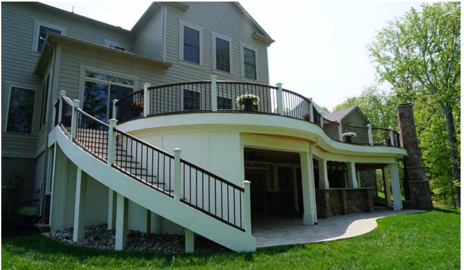
ABOVE: TREX TRANSCENDS DECKING AND RAILS: DRY UNDER SPACE WITH FINISHED CEILING, BAR, PATIO AND FULL MASONRY FIREPLACE. WHITE PVC TRIM AND PANELS. PAVER PATIO AND RIVER ROCK UNDER STAIRS.
