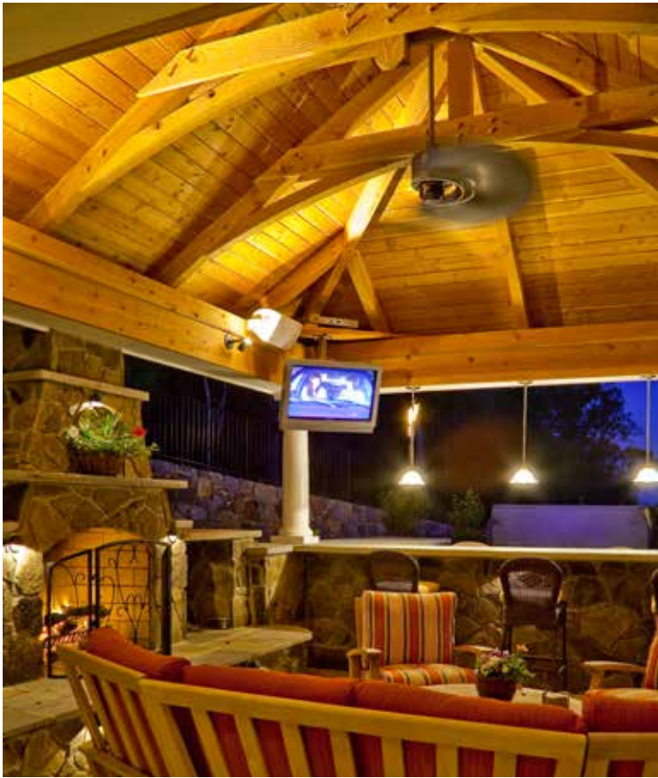
ABOVE: 10" round columns with white PVC trim. Holloway fieldstone seating bar and fireplace. Timber rafters.
