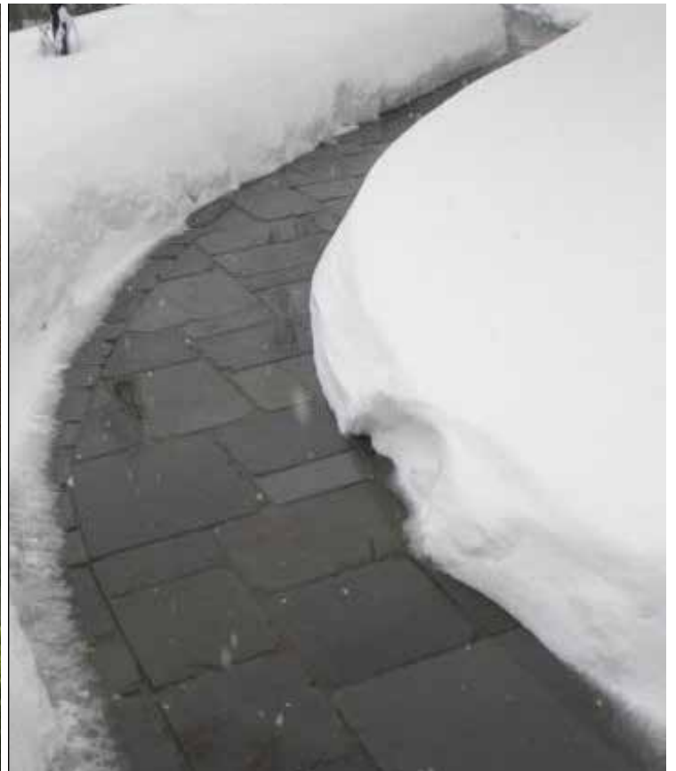
TUMBLED FLAGSTONE IN DRY BASE HEATED FOR ICE MELT.
