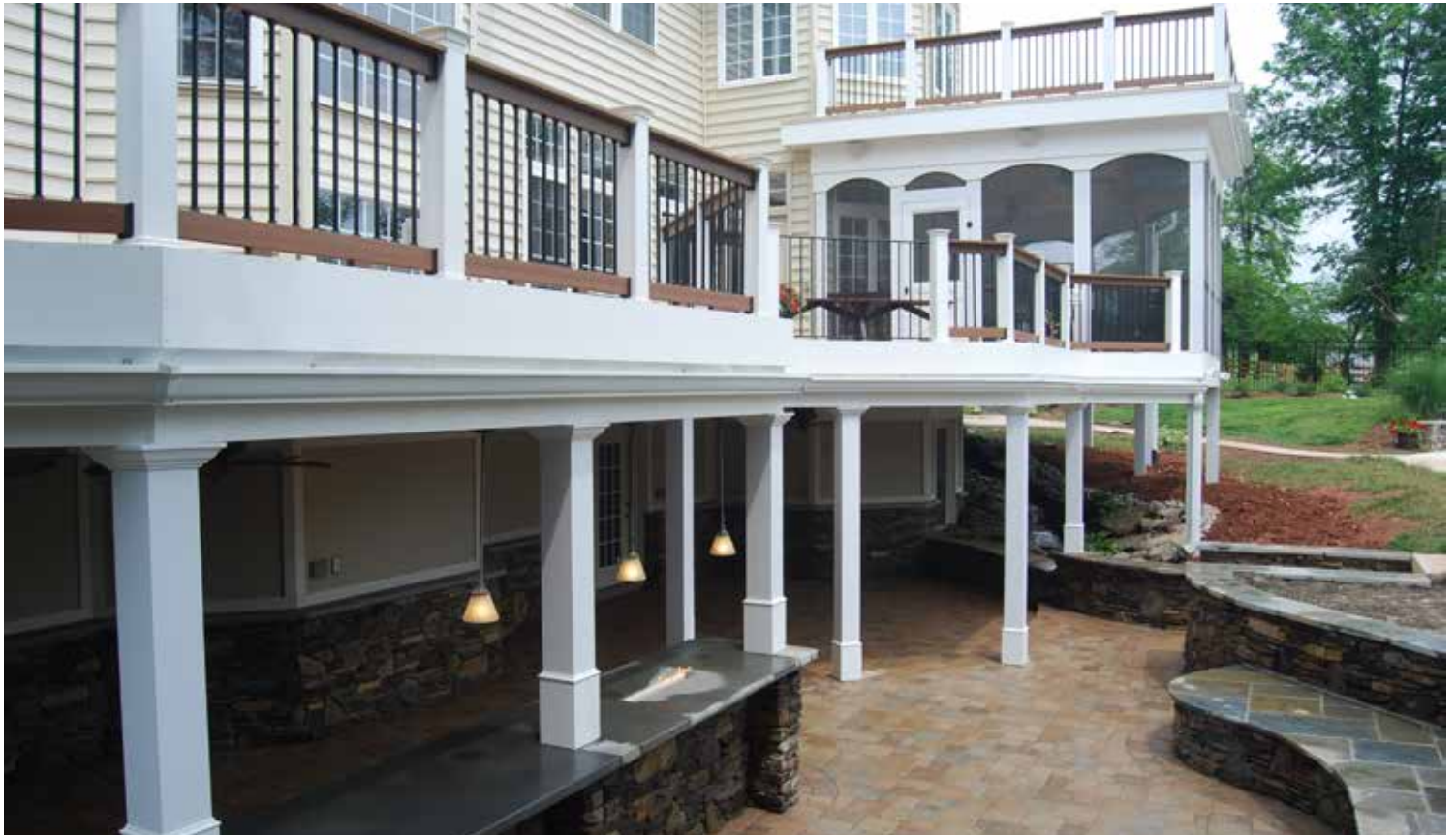
ABOVE: DOUBLE LEVEL DRY SPACE DECKS, COMPOSITE DECKING AND RAILS, WHITE PVC WRAPPED POSTS, ARCHES AND BEAMS. SCREENED PORCH, LOWER PATIO, BAR, FOUNDATION COVERED WITH 42" WATER-TABLE STONE AND HARDIE-BOARD ABOVE.
