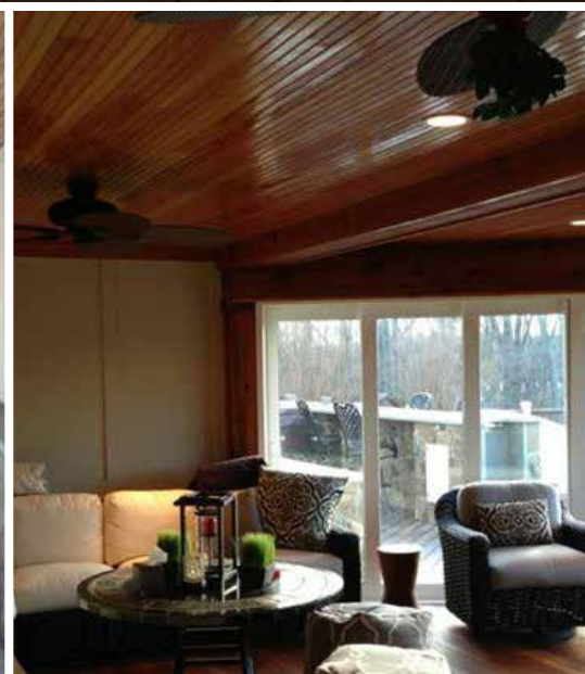
FINISHED BEADED FIR CEILING UNDER DECK WITH FOUR TRACK GLASS SLIDING DOORS
