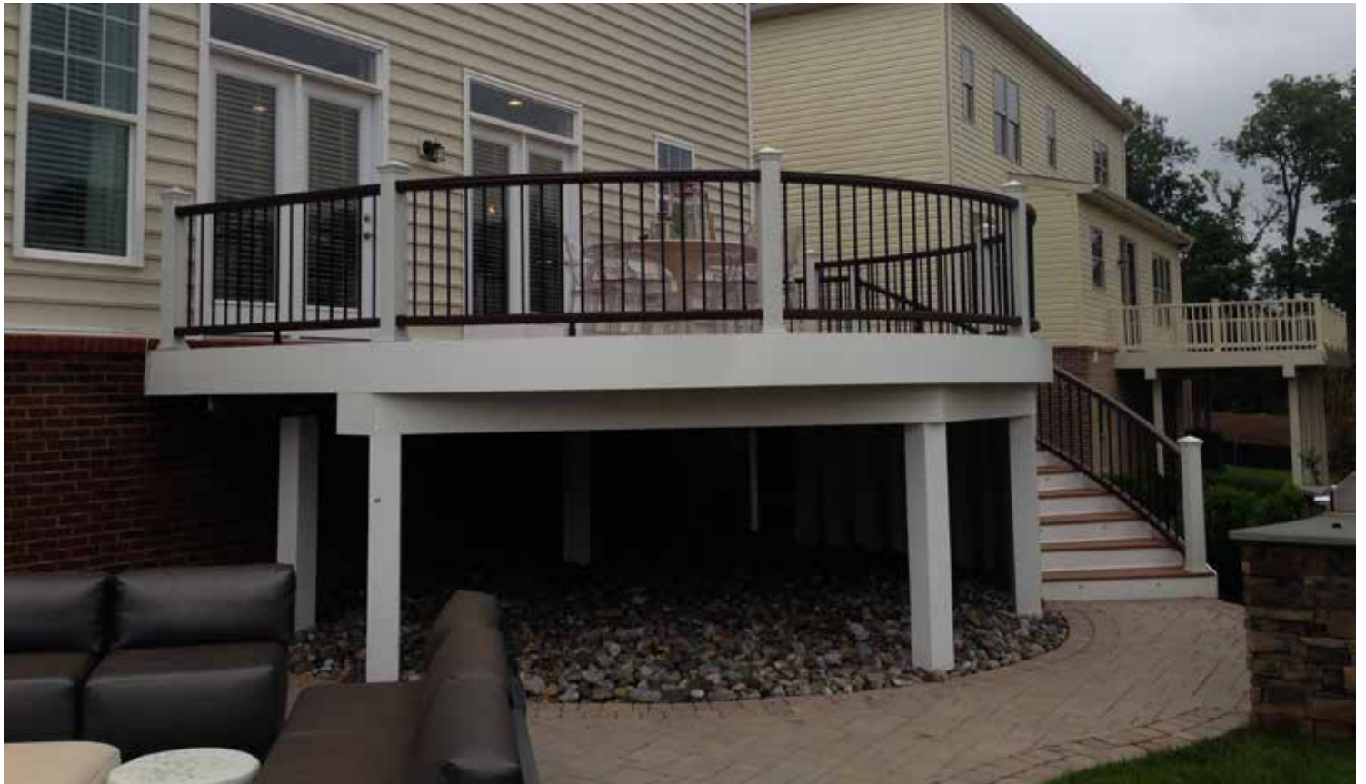
ABOVE: TREX TRANSCENDS CURVED DECK AND RAILS: VINTAGE LANTERN RAIL, WHITE POSTS, BLACK ALUMINUM BALUSTERS. RIVER ROCK UNDER DECK AND PAVER PATIO LEADING TO AN OUTDOOR KITCHEN.
