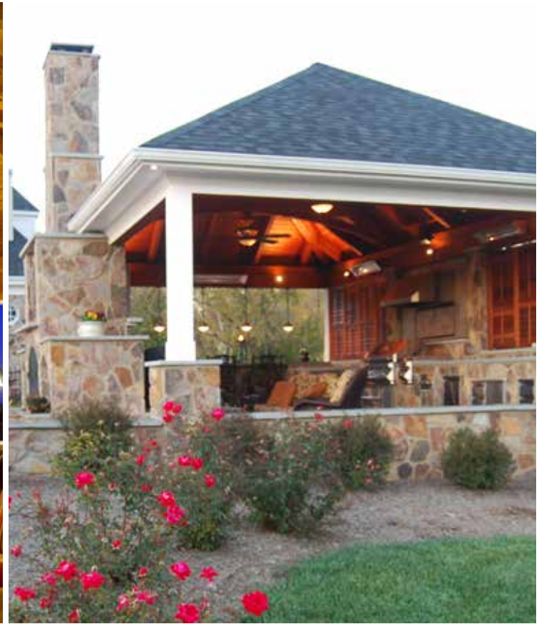
ABOVE: PAVILION. SEE THRU FIREPLACE WITH WOOD STORAGE. KITCHEN, BAR AND INFRARED HEATERS.
