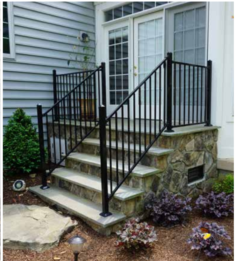
HOLLOWAY FIELDSTONE VENEER WITH FLAGSTONE TREADS AND ALUMINUM RAILS
