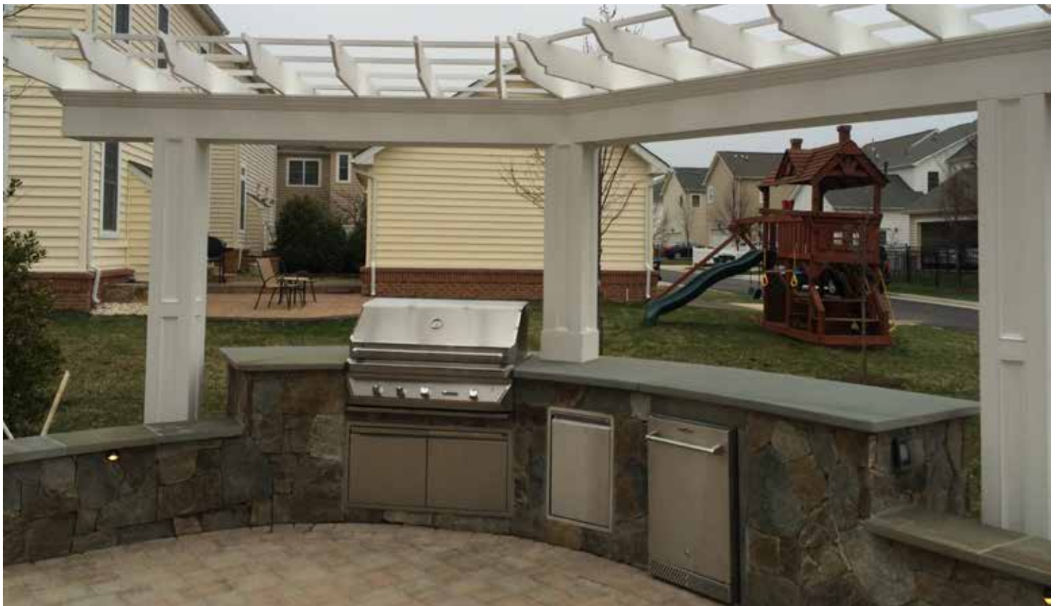
ABOVE: OUTDOOR KITCHEN WITH HOLLOWAY FIELDSTONE VENEER WITH BLUESTONE COUNTER TOPS, BUILT-IN GRILL, CABINETS, TRASH DRAWER AND REFRIGERATOR. HANOVER PATIO: CHISELED FINISH 50/50 MIX CHOCOLATE TAN AND SOUTH MOUNTAIN SAND.
