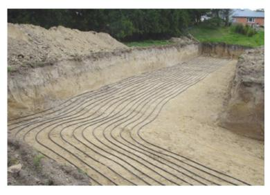
bottom of a wider trench. The trench lengths are likely to be 20-30 percent of the length of a single pipe configuration, but the pipe length may double for the same thermal performance.
