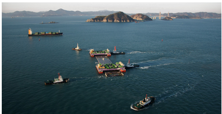
Fig. 10 Transport and immersion Busan Geoje (Photo Mergor)
