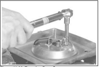
Figure 11-90. Torquing Base Screws.
