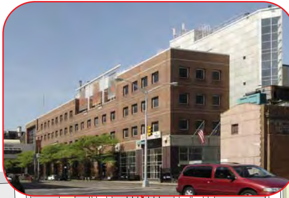
Building A: 475 Grand Concourse
