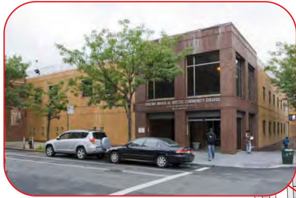
Building D: Savoy Building
