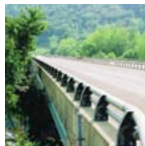
Athens Bridge - Pennsylvania.
