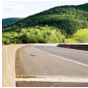
Tioga Bridge - Pennsylvania.
