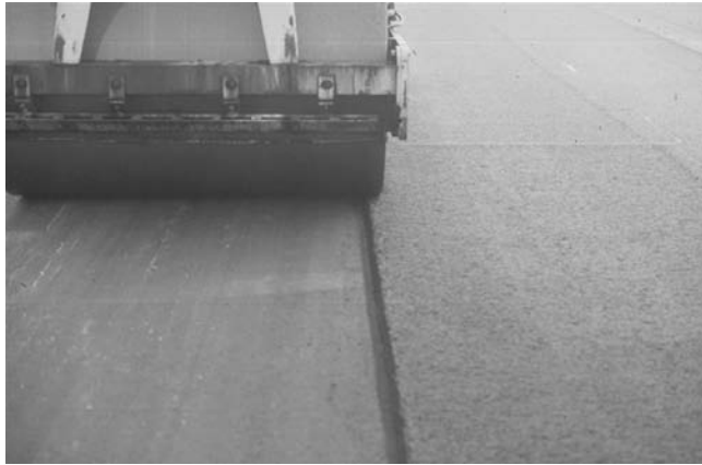
FIGURE 17-14 Starting compaction of longitudinal joint from the cold side, no longer a recommended practice.
