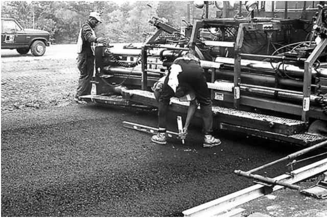
FIGURE 16-11 Checking slope of mat surface behind paver.
