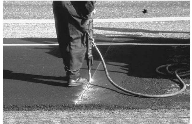
FIGURE 17-2 Removal of material at butt joint.
