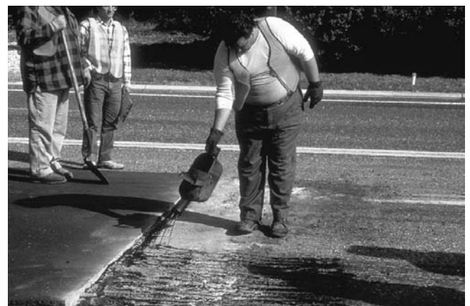
FIGURE 17-3 Application of tack at butt joint.
