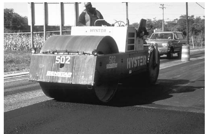
FIGURE 17-10 Longitudinal rolling of transverse joint.
