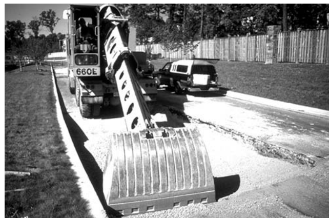
FIGURE 14-2 Removal of existing pavement prior to patching.
