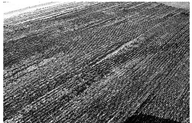
FIGURE 14-6 Tack coat on milled surface.
