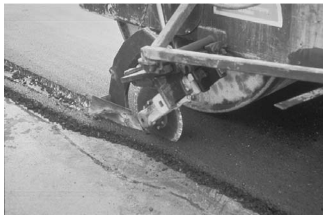
FIGURE 17-11 Cutting wheel used to construct longitudinal joint.
