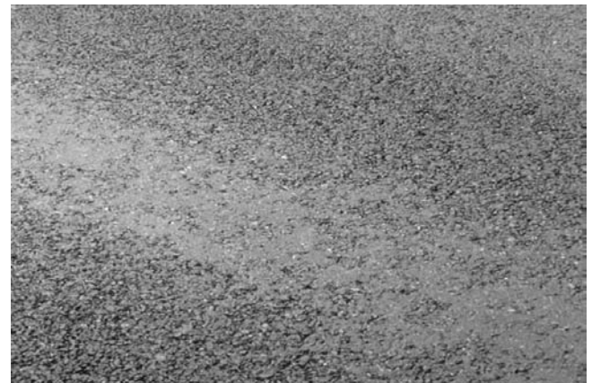
FIGURE 19-1 Nonuniform mat texture after compaction.
