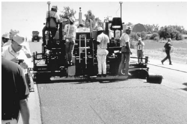
FIGURE 17-17 Compaction of mix in wedge joint.
