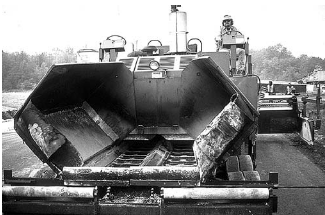
FIGURE 15-4 HMA paver with wings lifted.
