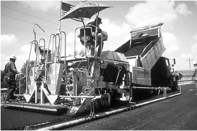
FIGURE 16-4 Paver with mobile reference employing rigid pipe.
