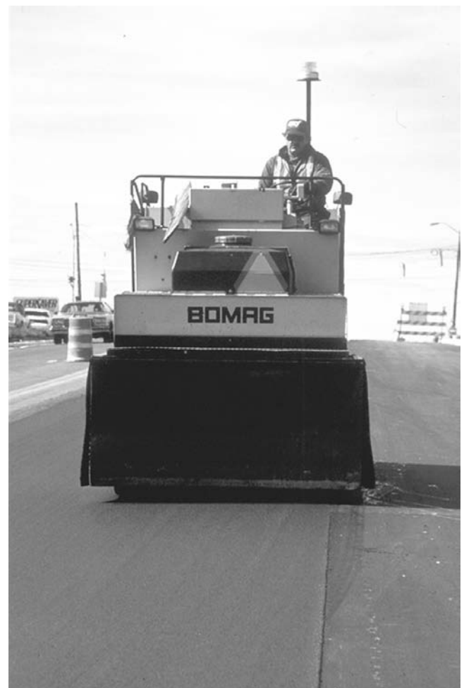
FIGURE 17-15 Compaction of longitudinal joint with pneumatic tire roller.
