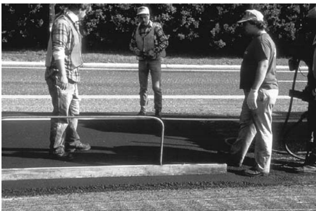
FIGURE 17-8 Checking smoothness at transverse joint.
