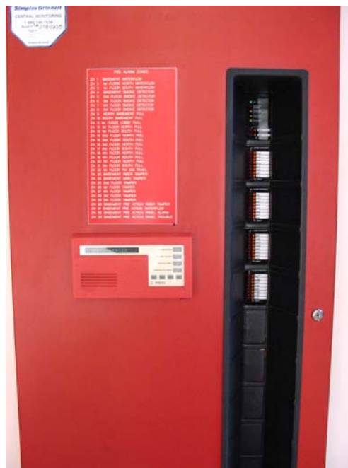
The presence of a trouble light does not necessarily mean that the alarm system is inoperative
