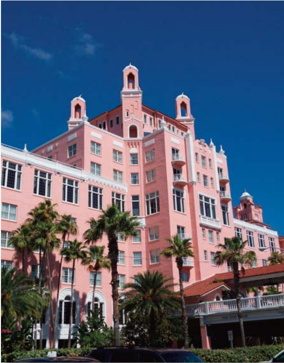
Hotels with prime locations and historically good occupancy, like the Loews Don CeSar Beach Resort in St. Petersburg, FL, pictured above, have been able to continue renovation projects as planned despite the economic downturn.
