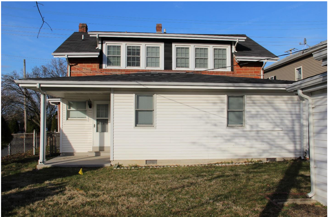
Figure 2: View of the east elevation from the rear yard. Photograph by Kyle Fisher, March, 2018
