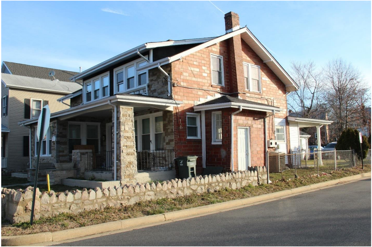
Figure 1: View of the south elevation from North Culpeper Street. Photograph by Kyle Fisher, March, 2018
