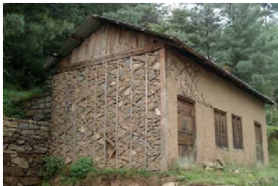
Figure 3 20. A dhajji building with gable wall with planks.
