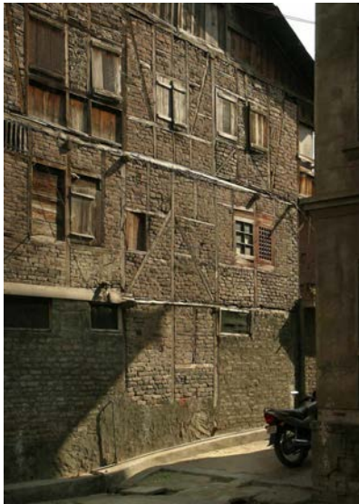
Figure 1 2. Multi-storey Dhajji building in Shrinagar, India. Photo source: © Randolph Langenbach.
