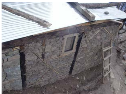
Figure 3 55. Mixed wall construction. Dry stone wall on the left hand side and dhajji construction on the right hand side. Note: The stone wall looks like it is against the slope; these are not strictly built as retaining walls, but as stone walls with loose fill behind.
