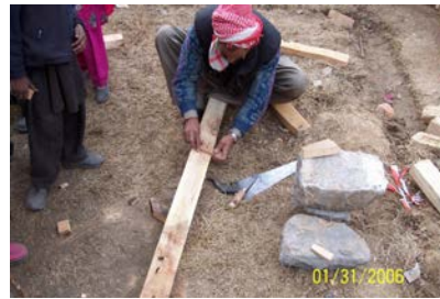
Figure 6 5. Improved tools to guide the carpenter made from scrap wood and nails on an ad hoc basis.
