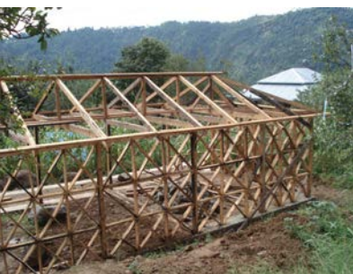
Figure 3 25. A view showing roof and braced timber frame.
