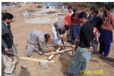
Figure 6 7. Cutting of timber sections. Note the child watching and learning.
