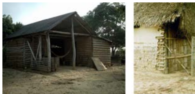
Figure 1 7. Examples of similar construction from Venezuela and South America: (left) Taquezal/Bahareque (source Wilfredo R. Rodríguez H.; Taquezal and Bahareque mean the same thing. Taquezal is the term used in Nicaragua, and Bahareque in El Salvador and other countries.), and (right) Quincha (source unknown).
