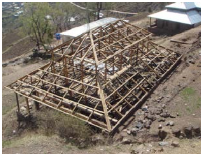
Figure 3 50. Double storey hipped roof built in to the slope on one side.
