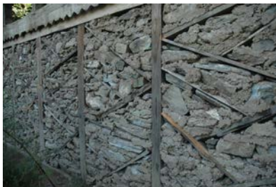
Figure 3 41. Wall built after the 2005 earthquake.
