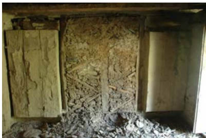
Figure 3 40. Wall built before the 2005 earthquake.
