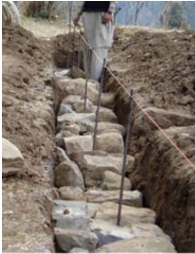
Figure 3 7. Bolts in the foundation to tie-up plinth timber.
