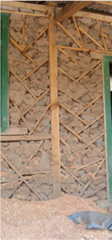
Figure 3 19. Herringbone bracing pattern.
