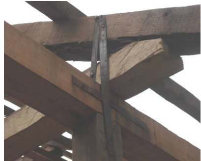
Figure 3 24. Tie-up of roof with wall structure.
