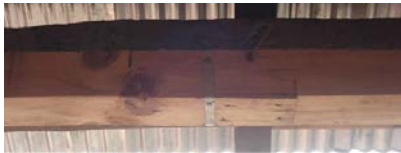
Figure 3 31. Simple strapping of nailed scarf joint will provide confinement to the joint and help increase its capacity. The nailing increases the scarf joints tensile capacity.
