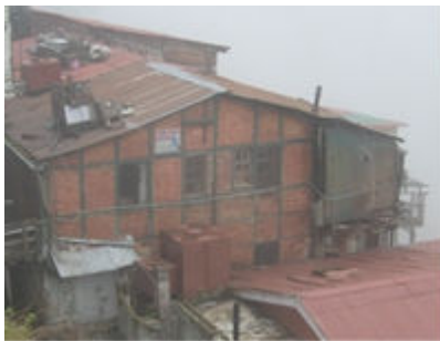
Figure 1 1. A Dhajji building in Simla, India without bracing elements.
