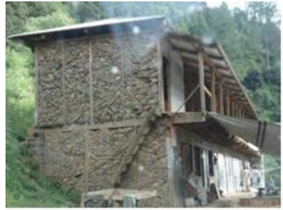
Figure 1 3. A two storey Dhajji building that survived the 2005 Pakistan earthquake whilst most buildings around it fell down.
