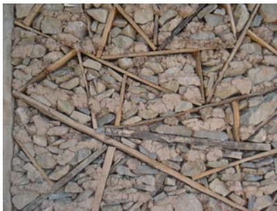
Figure 3 34. Common random bracing in small panels.
