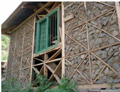
Figure 3 35. X-bracing pattern using partially cut stone.
