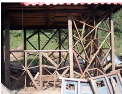
Figure 3 26. Mixed bracing pattern making use of salvaged timber and window frames.
