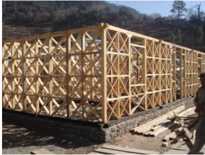
Figure 3 43. Engineered dhajji building frame under construction.
