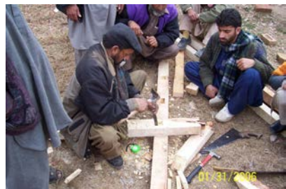
Figure 6 6. Hammer, chisel and saw are the main tools to construct a dhajji house.
