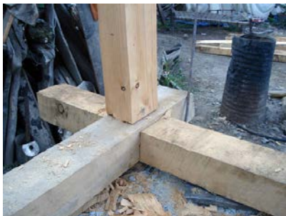
Figure 3 10. Corner connection detail with generous overlaps.
