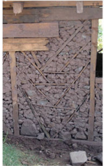
Figure 3 18. Inverted A-bracing pattern.
