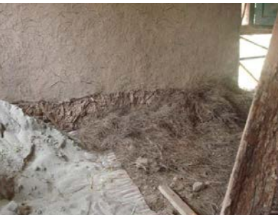
Figure 2.7. Plastering with cement sand plaster or mud mixed with natural fibres.
