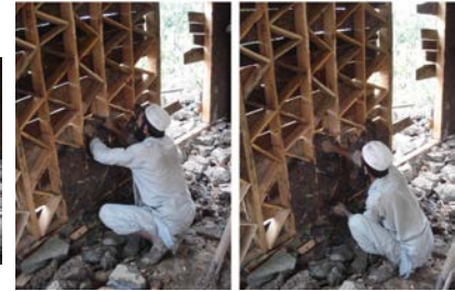
Figure 6 12. Construction of the infill walls continued.
