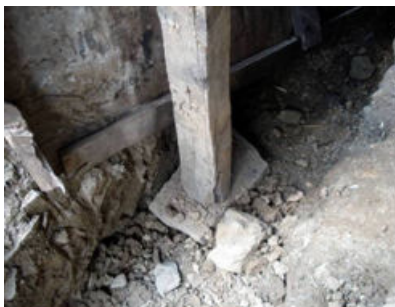
Figure 5 23. Example of effort to provide foundation to a timber post to reduce the immediate settlements under the post and provide limited protection to the timber end grain from moisture.
